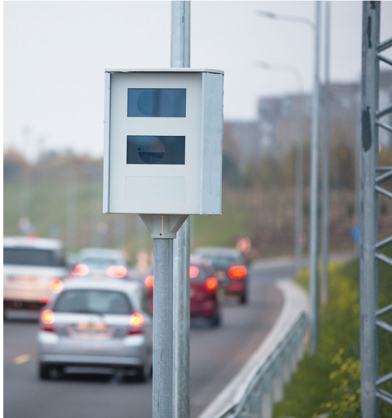
Drivers at Vilnius Western Bypass are controlled by four speed meters.
